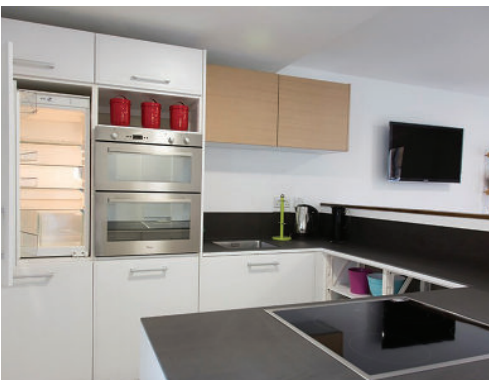
Resilient kitchen with raised appliances and power sockets. Tiled floors and kitchen units can be cleaned and dried
