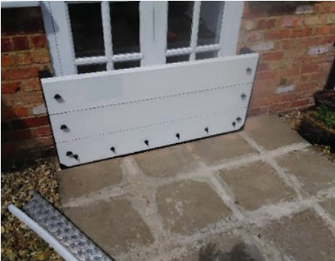
Door flood barrier manually fitted to reduce the entry of flood water
